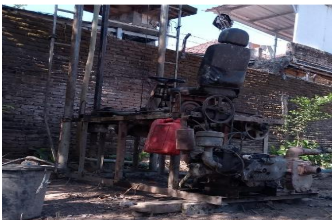
Gambar 1. Pengeboran Sumur Bor ( Deep Well )
